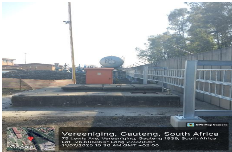
Figure 11: Site Observations: The Start of the Final New System
