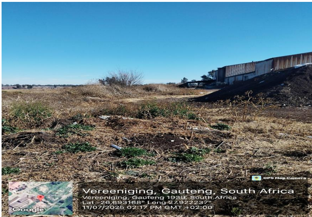
Figure 15: The pipeline continues traveling underground into private property, specifically within the yard of a private residence or facility.
