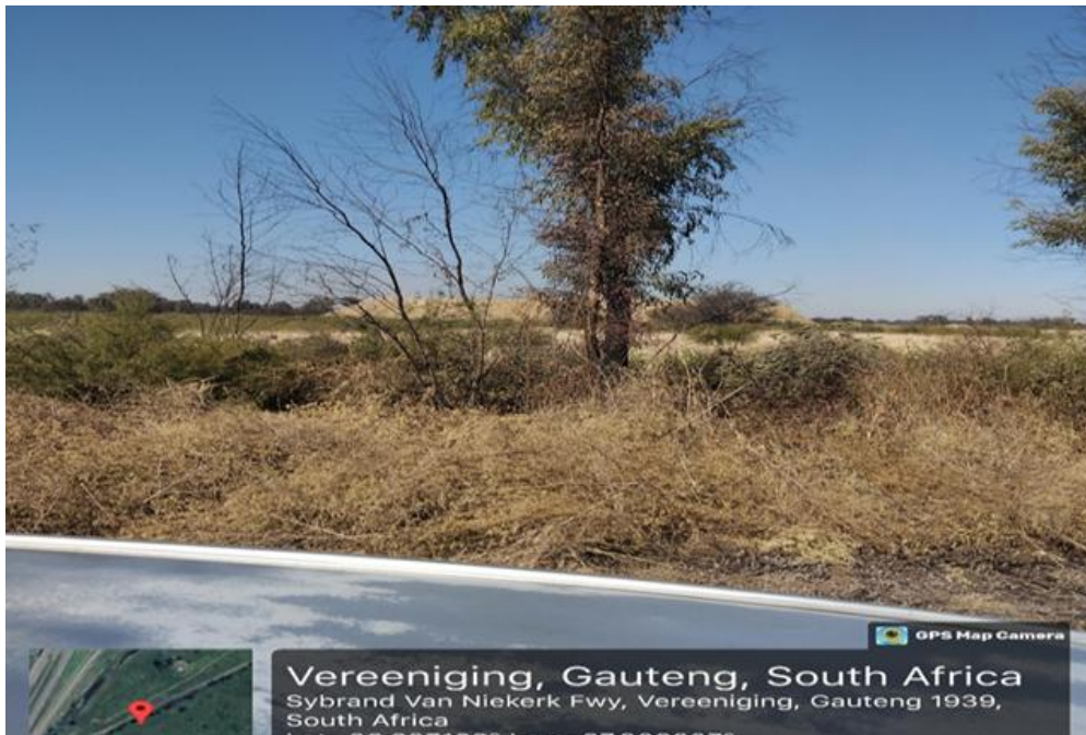
Figure 14: Sludgeline Phase 2 pipeline crosses under Barrage Road from Rand Water VG property to the other side.
