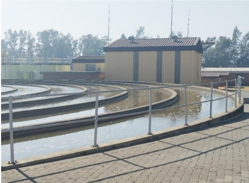
Figure 12: View of the existing flocculators at Vereeniging treatment Works.
